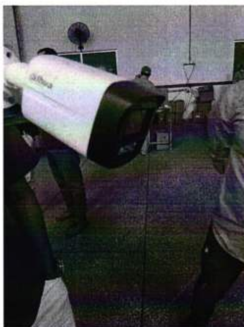
Image 2 — Dahua surveillance camera installed by the Vendor on the production floor
