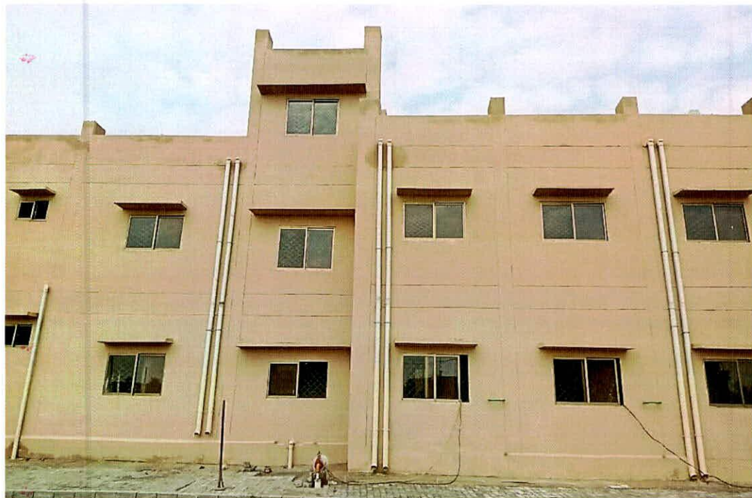
Rear Side View of Zonal Office Building
