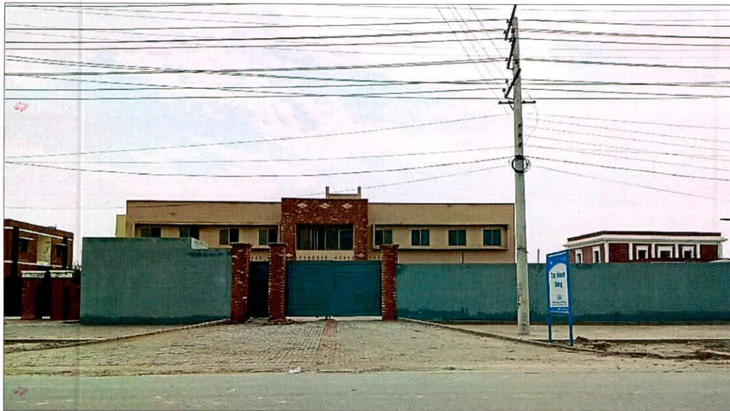
Front View of Zonal Office Building
