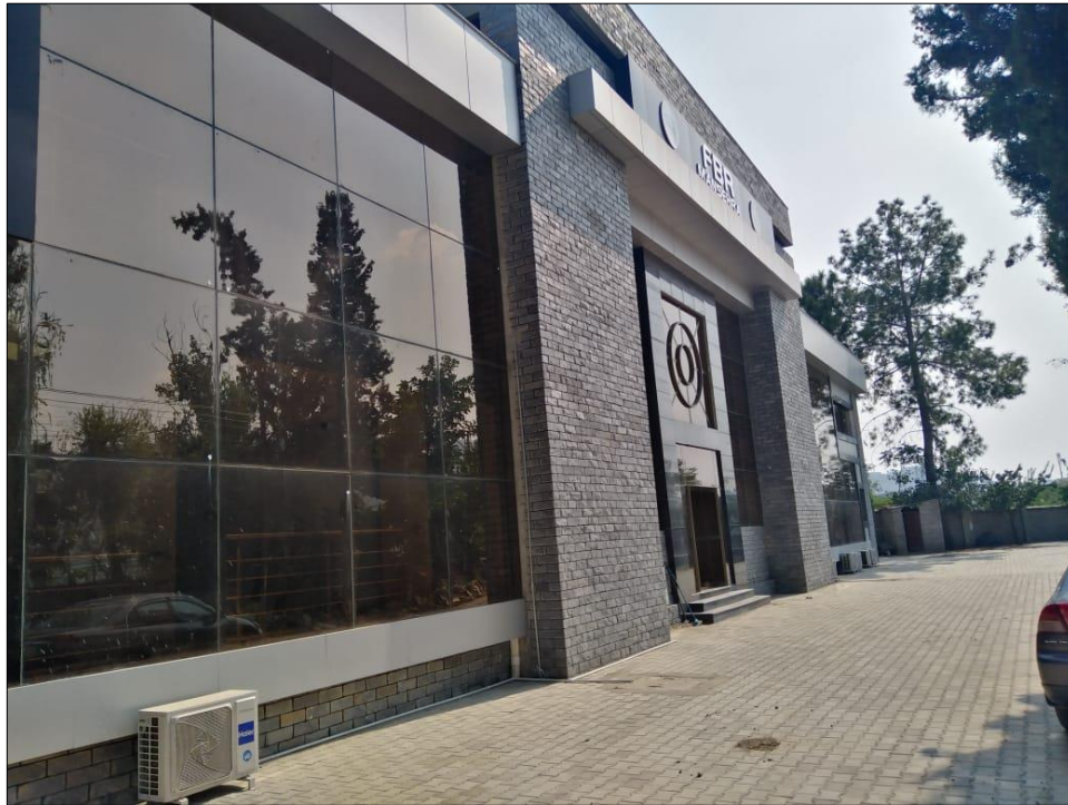
Side View of Zonal Office
