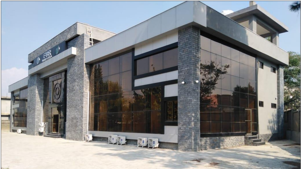
Front View of Zonal Office
