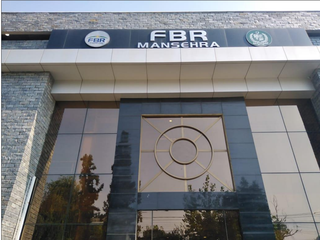
Front View of Zonal Office
