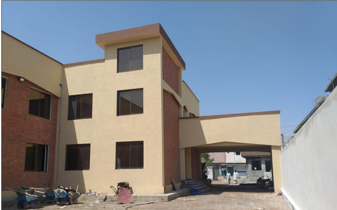
Front View of Zonal Office
