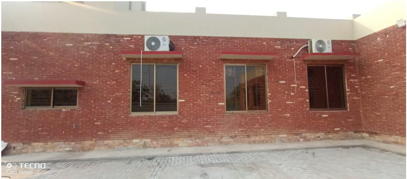
Windows View of IRO Building
