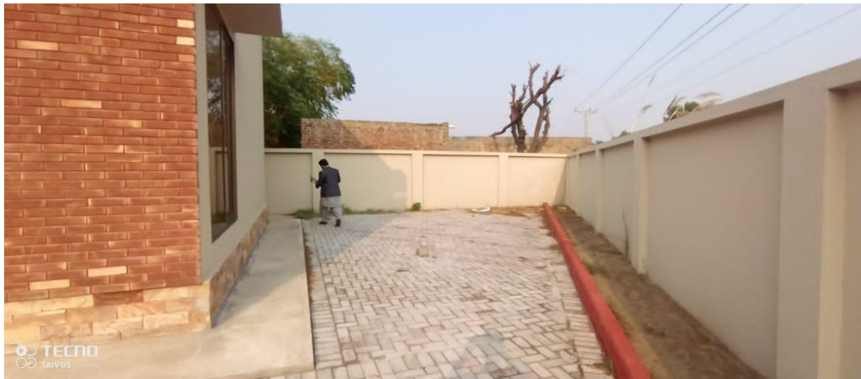
Boundary Wall of IRO Building
