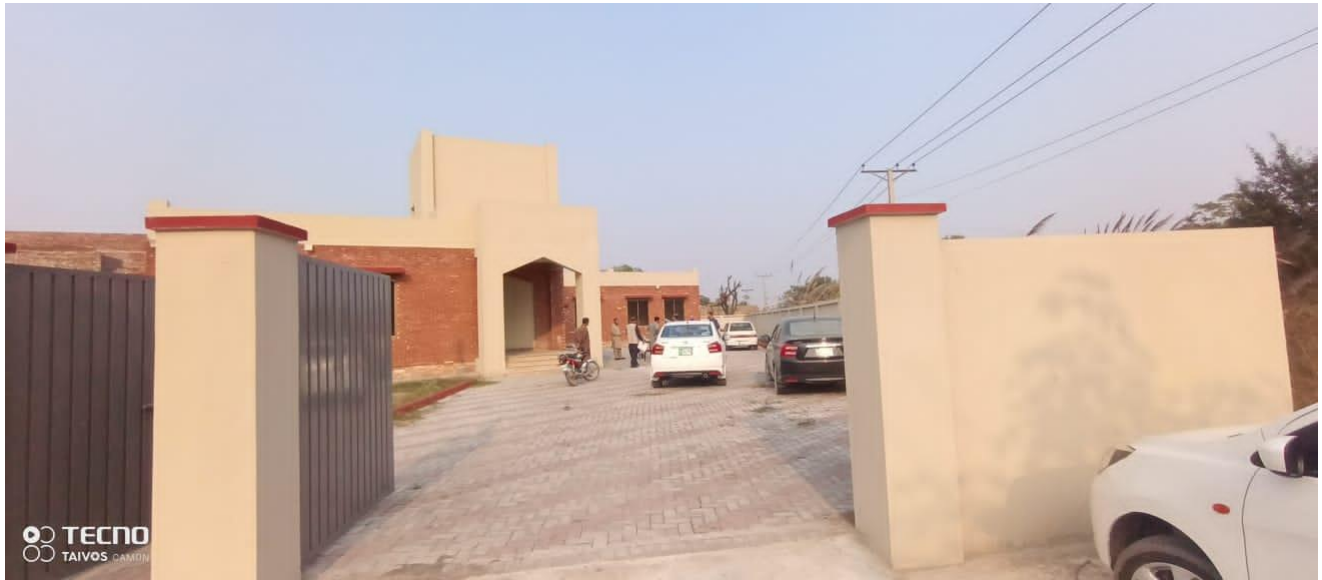
Front View of IRO Building
