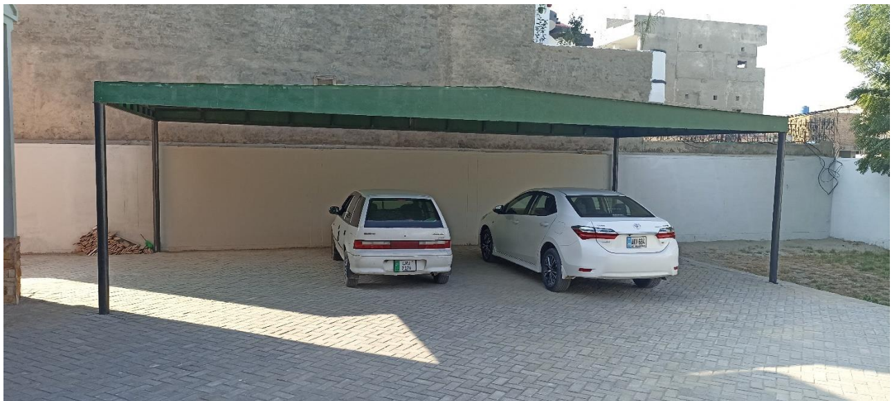
Parking Shed View of IRO Building
